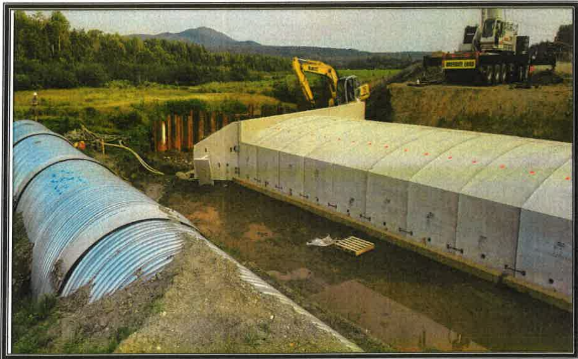
Knowles Flat Culvert Replacement
